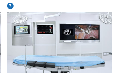
Shanghai No. 10 People's Hospital Shanghai, China
